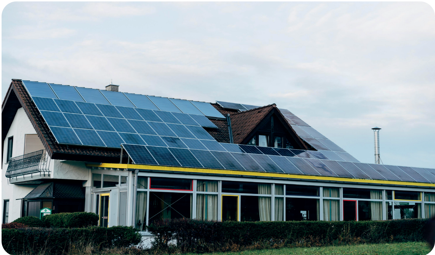
Solar panels harness renewable energy from the sun.
